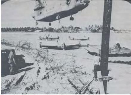
CH-47 EMPLACING AIRMOBILE FIRING PLATFORM
